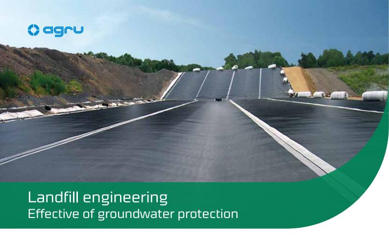
The sealing system is chosen depending on the materials stored at the landfill. In some cases, a second layer of HDPE or LLDPE geomembranes is even used alongside other geosynthetics. However, the geomembrane is always the primary sealing element at a landfill, to prevent rainwater from penetrating when the surface of the cell is being sealed, and to prevent groundwater from being contaminated via the cell's base seals.
